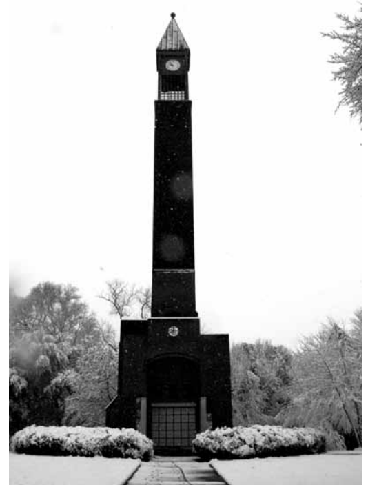
Millsaps Tower, February 2010
