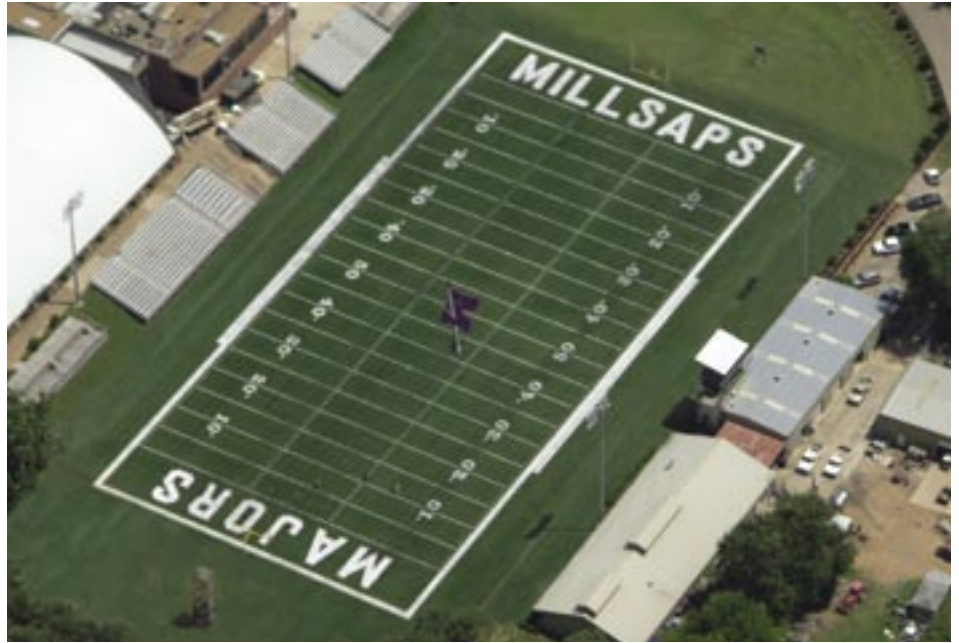
An aerial photograph of Alumni Field, which has been refitted with Sprinturf, a state-of-the-art artificial surface.
